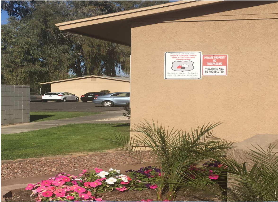
655 S. Magnolia Ave. 32 units 1,2,3 bedrooms, Yuma Police Substation, Crime Free Zone
